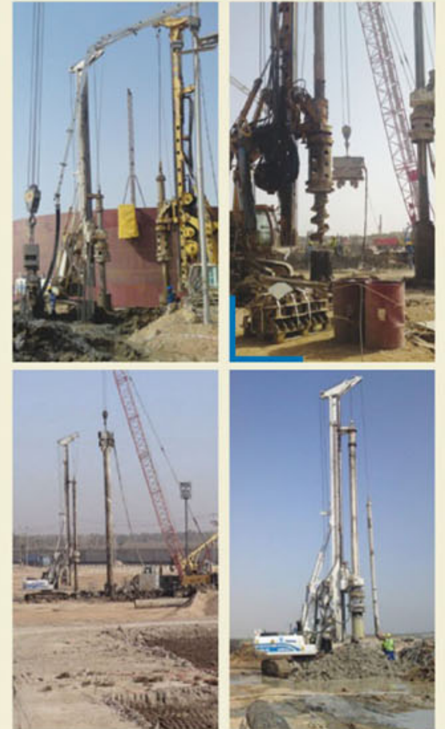
AL-KHAIRAT 1250 MW GAS POWER PLANT PROJECT, KERBELA-IRAQ
