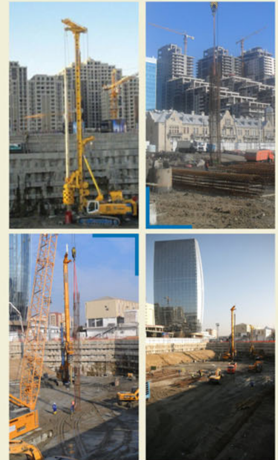
CRESCENT DEVELOPMENT PROJECT, BAKU-AZERBAIJAN
